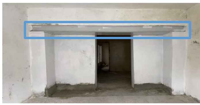
Figur 2, Steel beam in opening, white house
